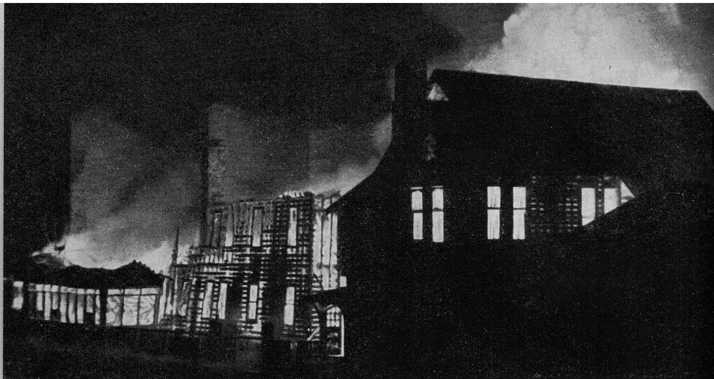
The Fire from the North Side.
